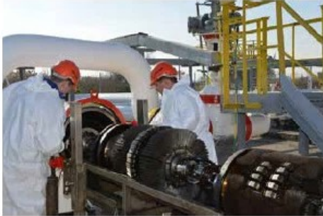
Figure 1. Launching of the combined tool on the client's pipeline system, Russia.
